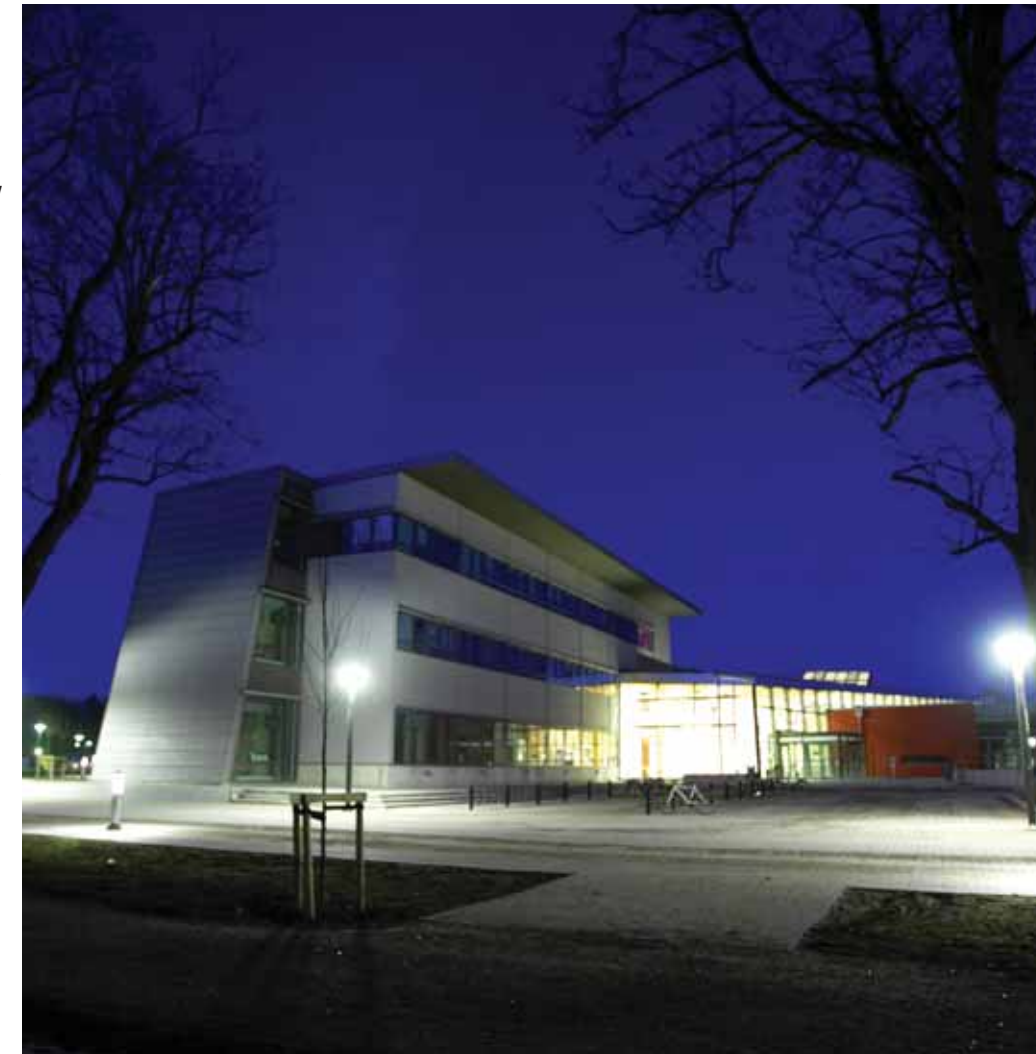
The Wood House at Växjö University. One of the largest multi-storied wooden buildings in Europe.
